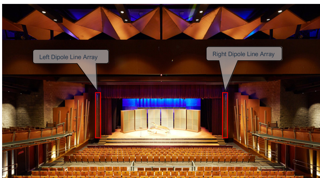
Figure 4 – View to Stage in Hall with Dipole Array Stage Left and Right
